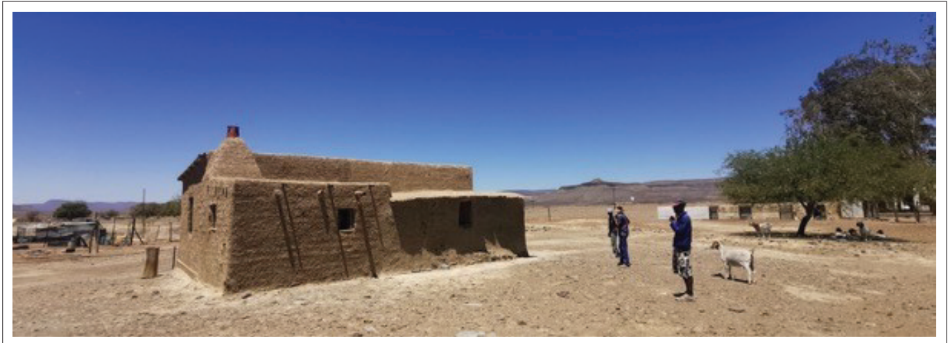
FIGURE 16: Jan Jollies' house viewed from the west. This façade needs regular re-plastering as it faces the direction from which the main stormy weather comes.
